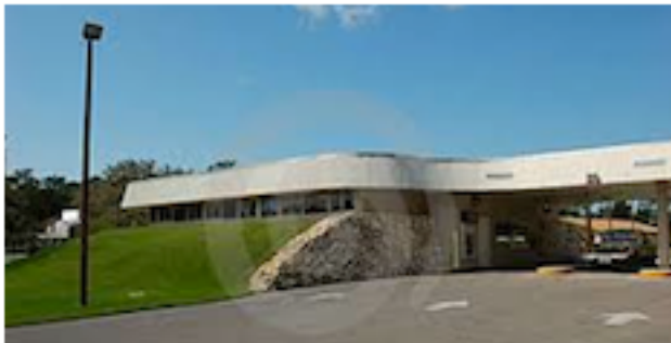
Bermed buildings: in these two, only the walls below window level are soil-insulated
