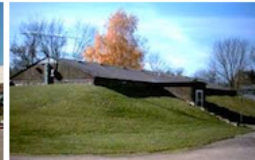
Bermed buildings: in these two, only the walls below window level are soil-insulated
