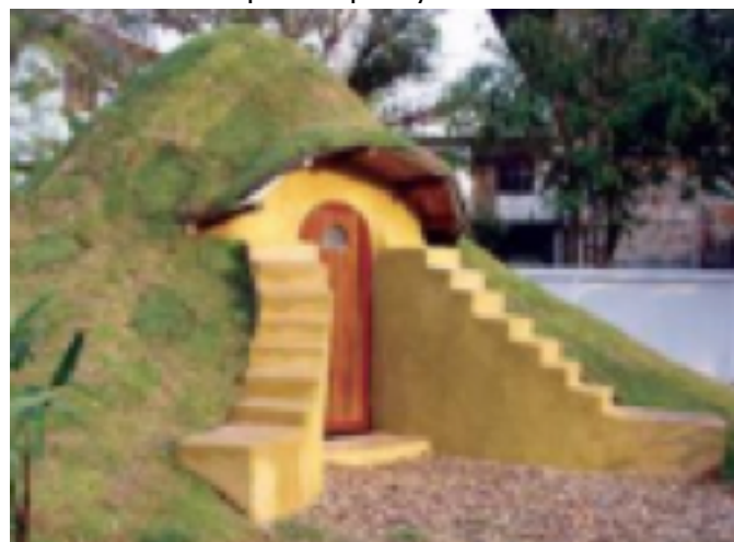
Necessarily exposed entrance to an “Earthbag” home http://earthbagplans.wordpress.com/introduction/
