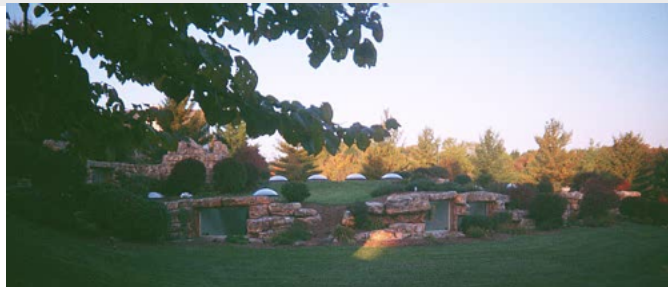
Photo of the exterior of Terra Lux taken twenty years later – The turning sun-facing cowls had been replaced by simple domes. The exterior window panes of three periscopic windows units are visible.
